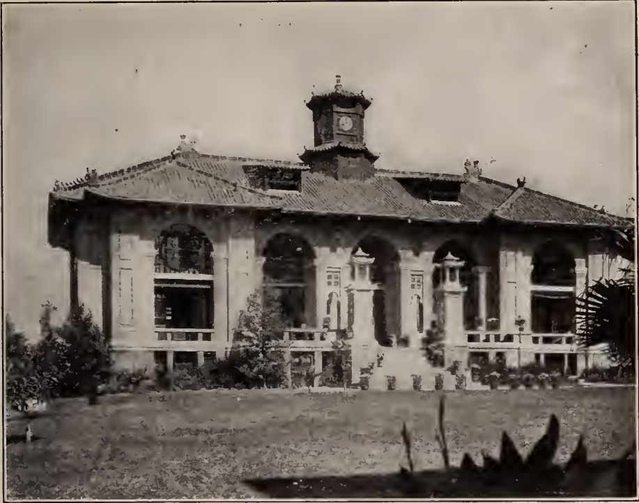
THE ADMINISTRATION BUILDING, CANTON CHRISTIAN COLLEGE
